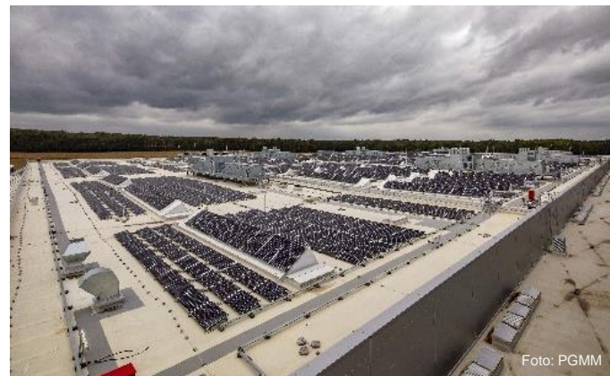
ACCUmotive Kamenz Expansion production site, Plant II
