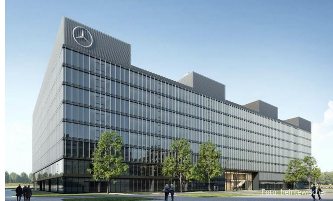
Daimler Sindelfingen New center for electric integration EIZ with test bench, body shop and administration
